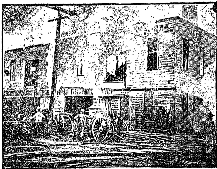
FRONT OF BUILDING WHEN FIRE WAS AT ITS HEIGHT.
