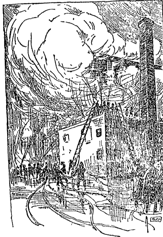
SCALING THE DRY HOUSE TO STREAM THE REAR OF THE WAREHAM STREET BUILDING.
