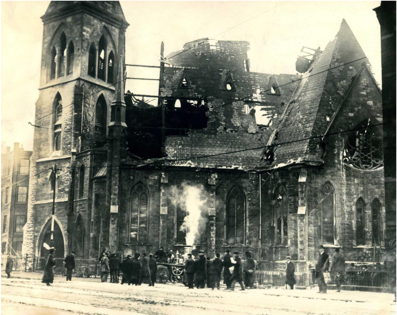
Second Universalist Church Fire, February 10, 1914. 65 Clarendon Street, South End, 4 Alarms, Box 80, 0053 Hours.
