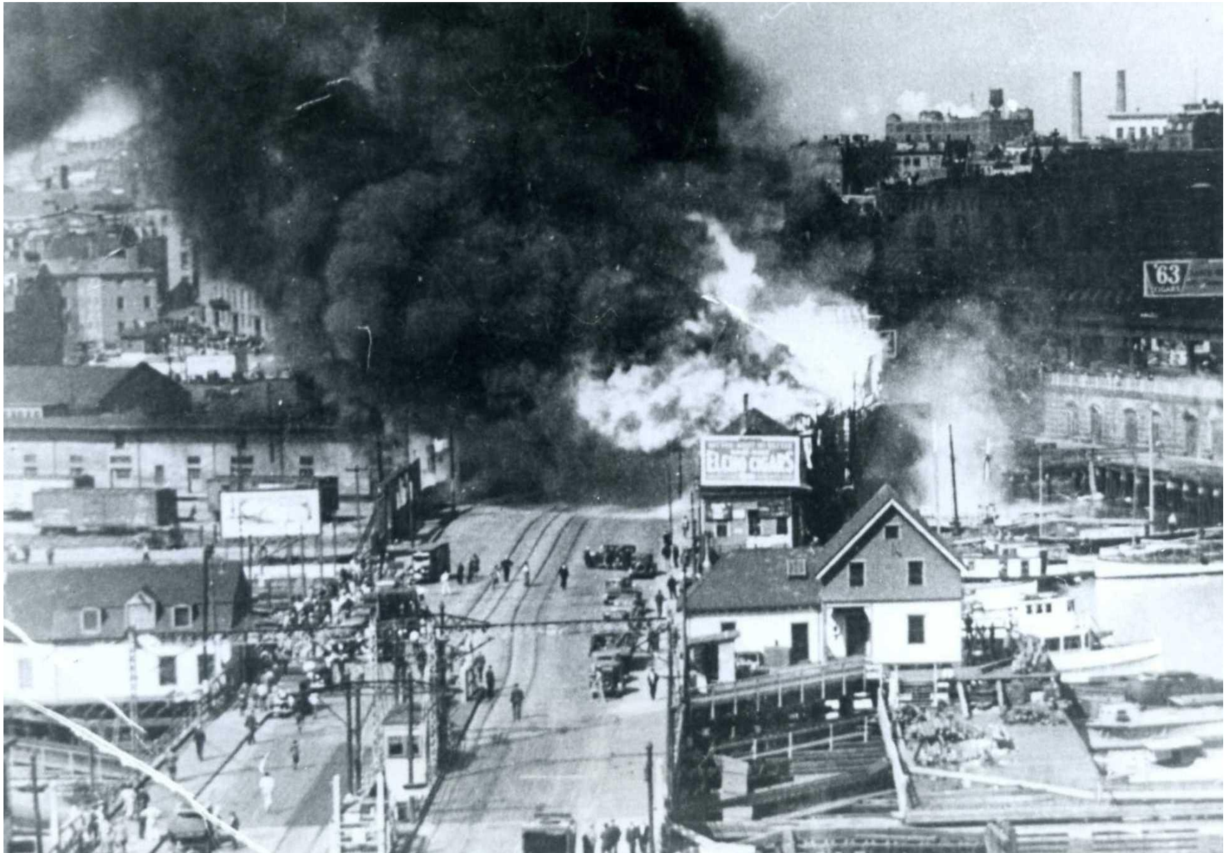
Buildings near Warren Avenue Bridge, September 24, 1935. 3 Alarms, Box 4112, 1345 Hours.
