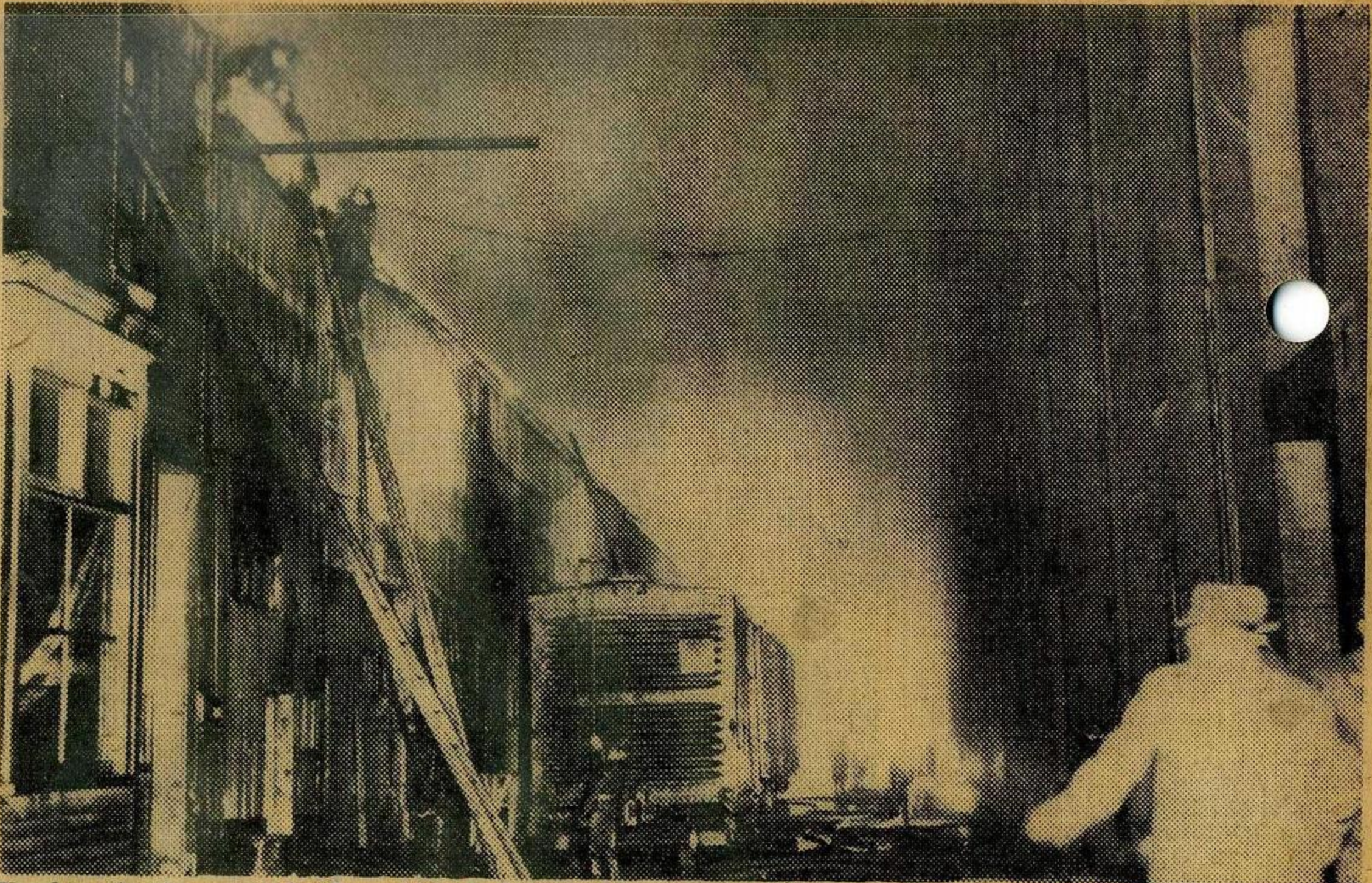
Wreckage in the wake of a fire which destroyed the warehouse of the Grasselli Chemical Company, 300 Congress street, South Boston, last night, injuring three firemen and causing damage of $100,000.
