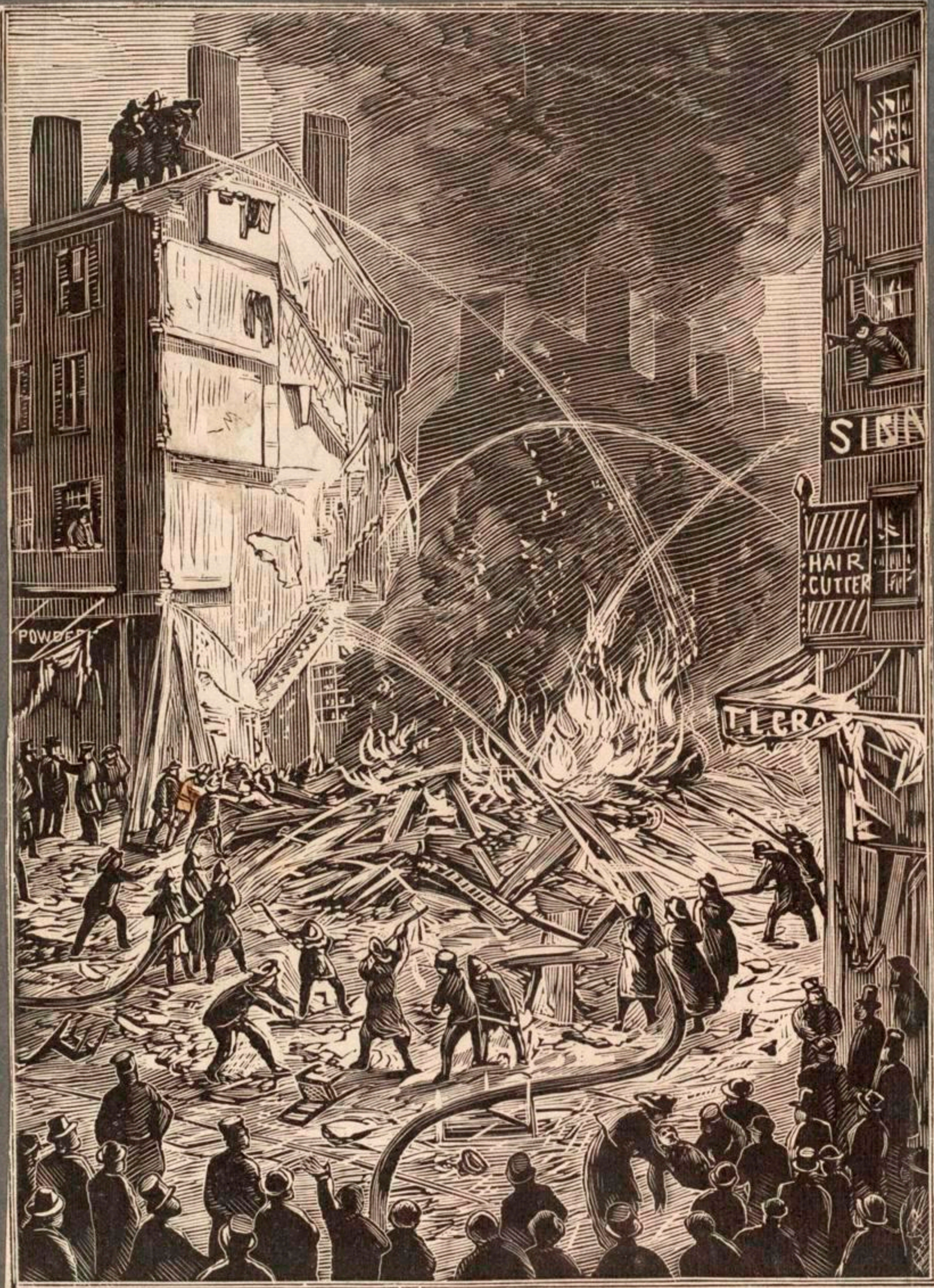
Scene after the terrible Explosion, cor. of Washington and Lagrange Streets, on May 26, 1875.
