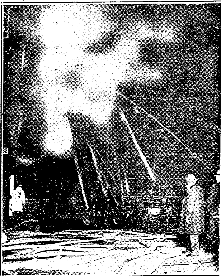
SCENE DURING THREE-ALARM FIRE ON LONG WHARF
