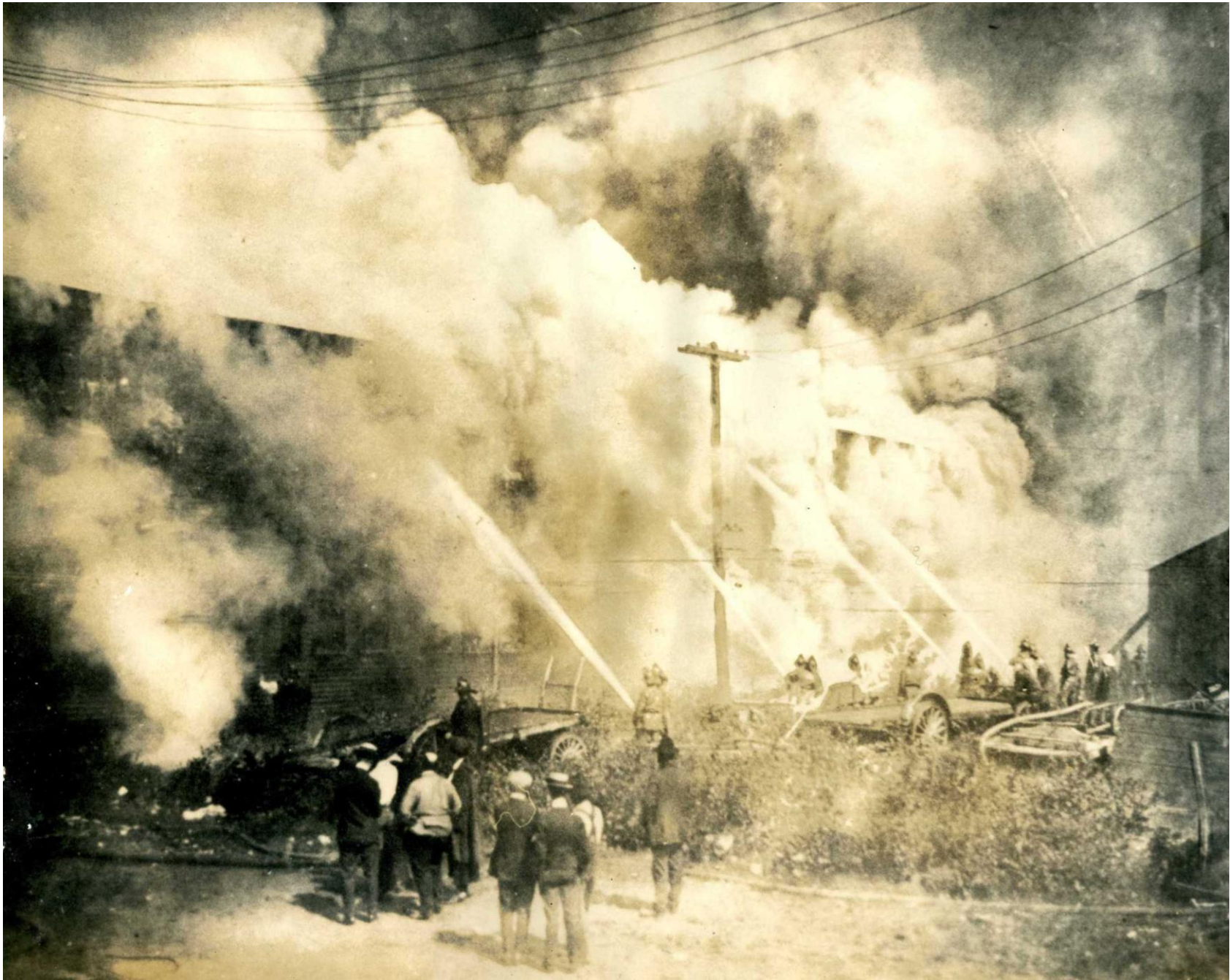
T. C. Ashley Company Fire, June 4, 1917. Rear 500 East First Street, at K Street, South Boston, 5 Alarms, Box 7323, 0830 Hours.
