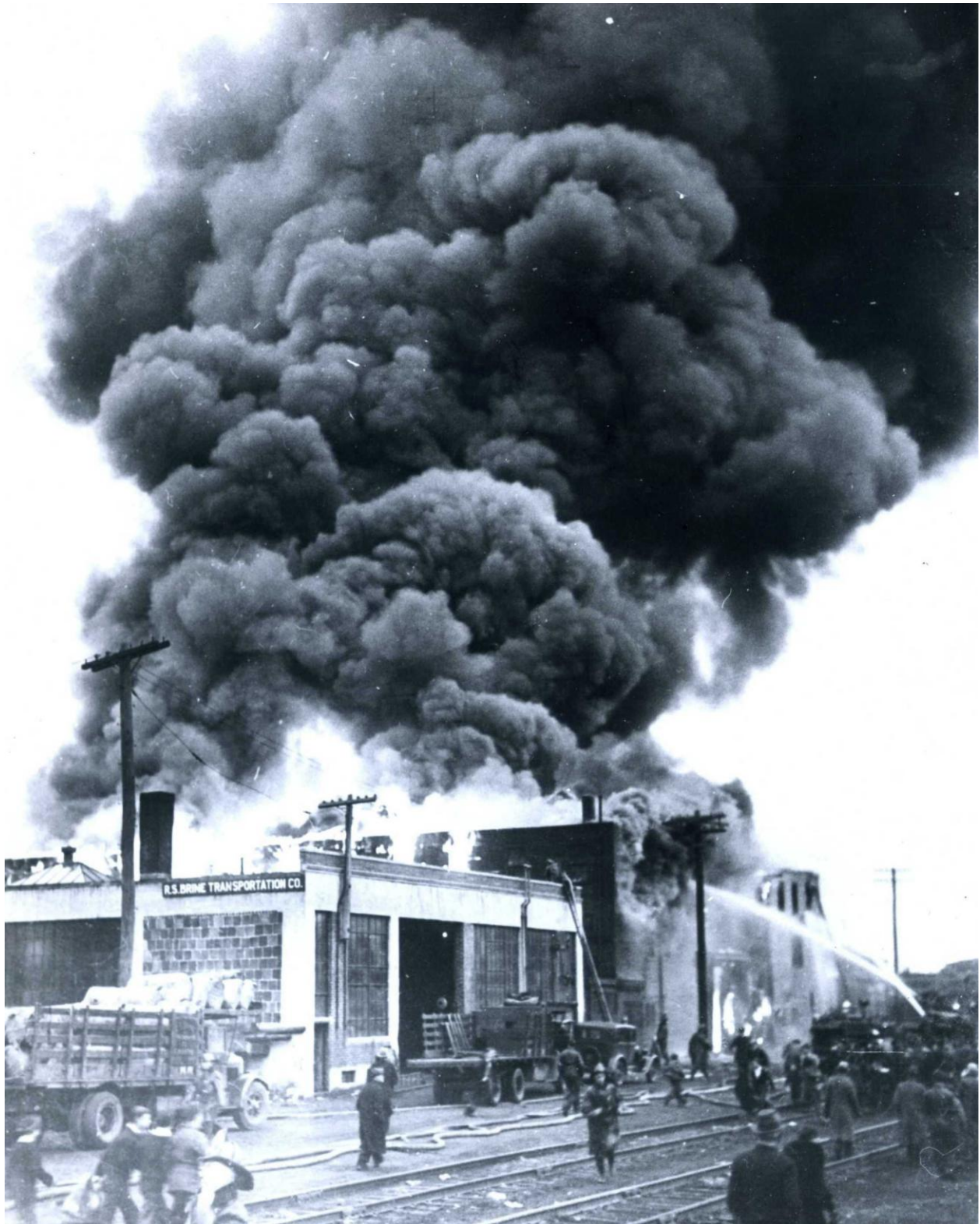
Cypher Street Fire, March 14, 1935. 15-17 Cypher Street, South Boston, 4 Alarms, Box 715, 1730 Hours.
