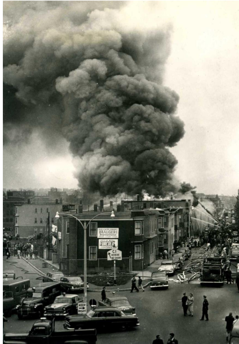
East Boston Fire, November 8, 1956. Saratoga, Curtis & Chaucer Streets, East Boston. 5 Alarms, Box 6213, 1304 Hours.
