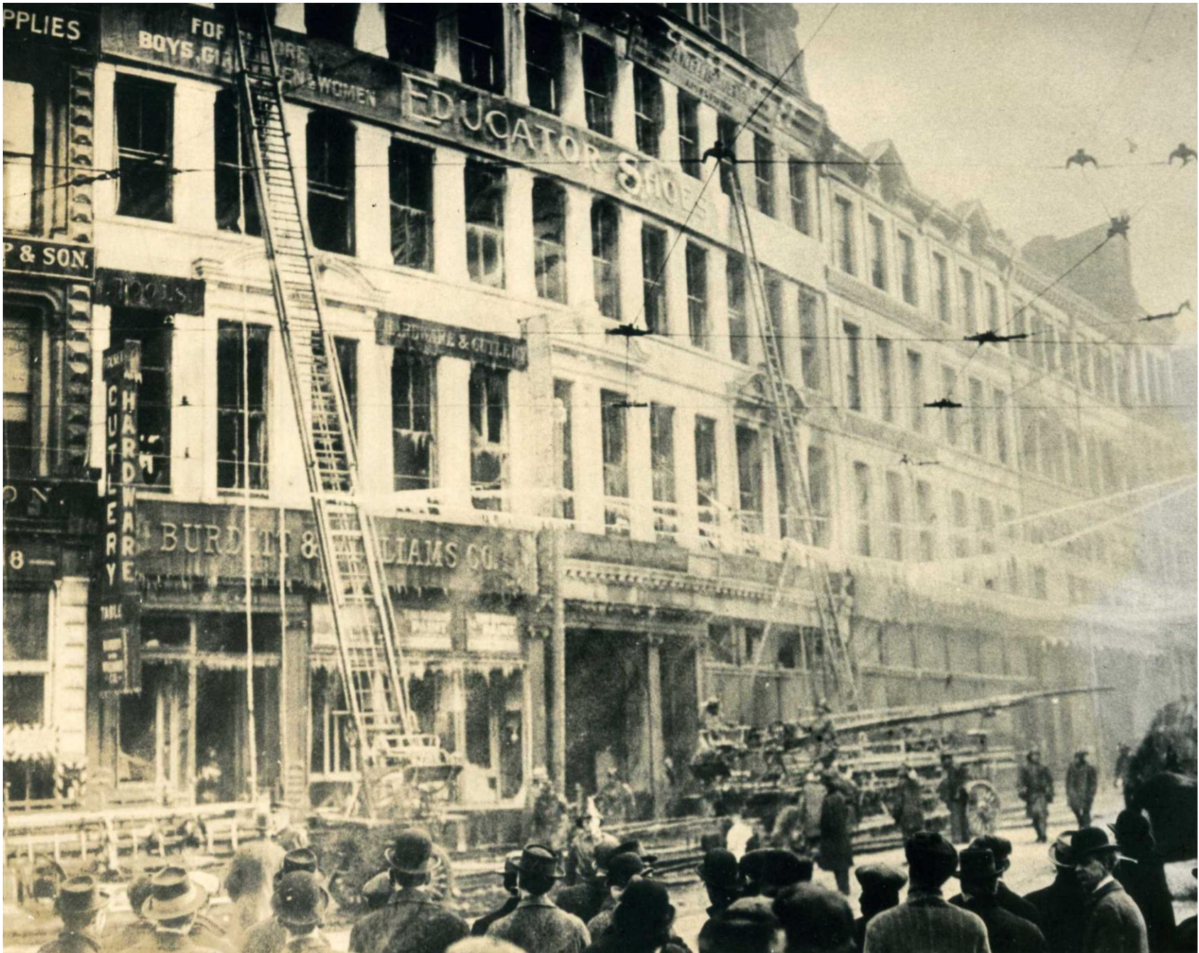
Rice Building Fire, March 3, 1915. 4-12 High Street, Downtown, 4 Alarms, Box 1431, 0102 Hours.
