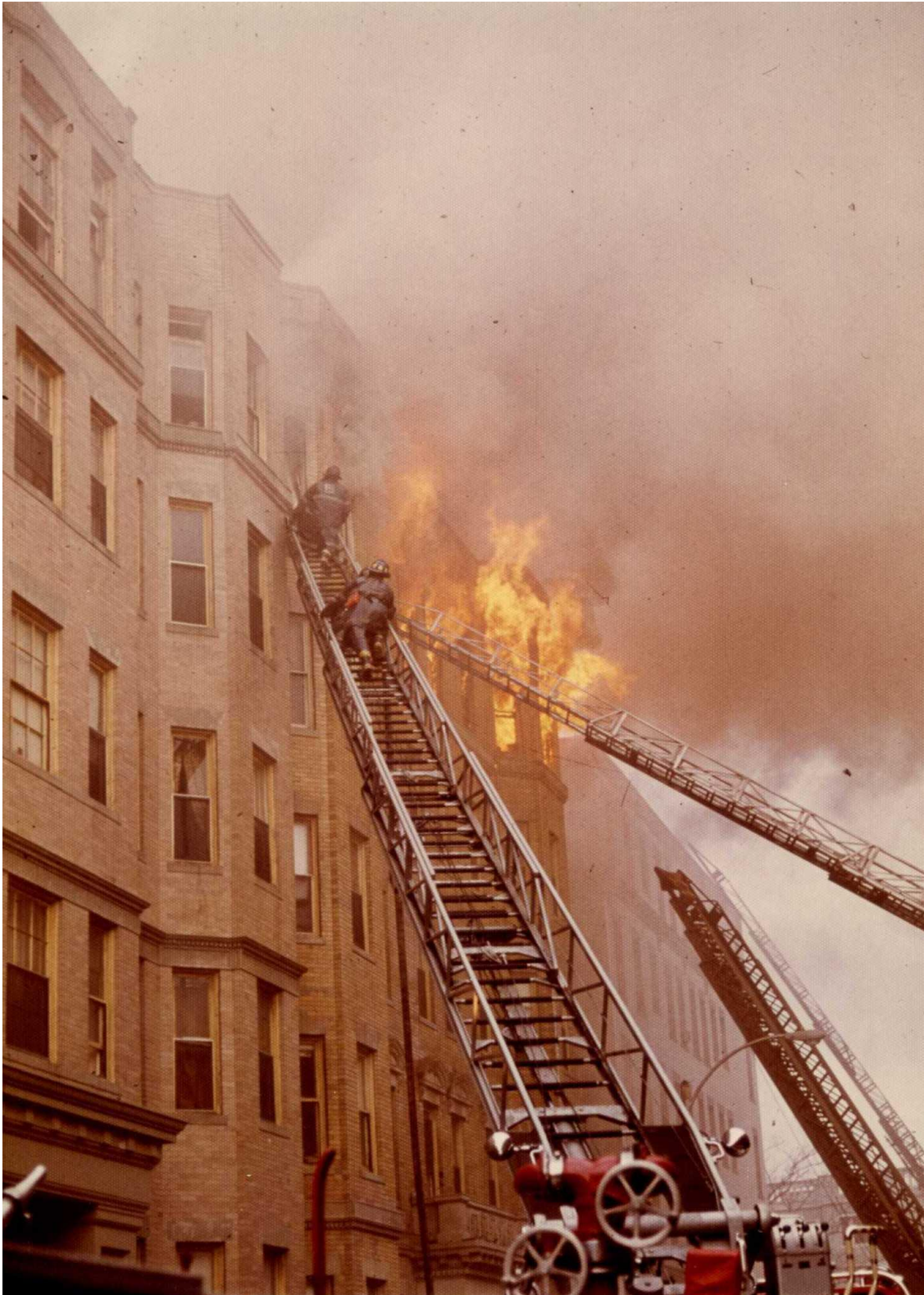
Royce Road, Allston, Fire, March 7, 1974. 5-11 Royce Road, Allston, 4 Alarms, Box 5143, 0759 Hours.
