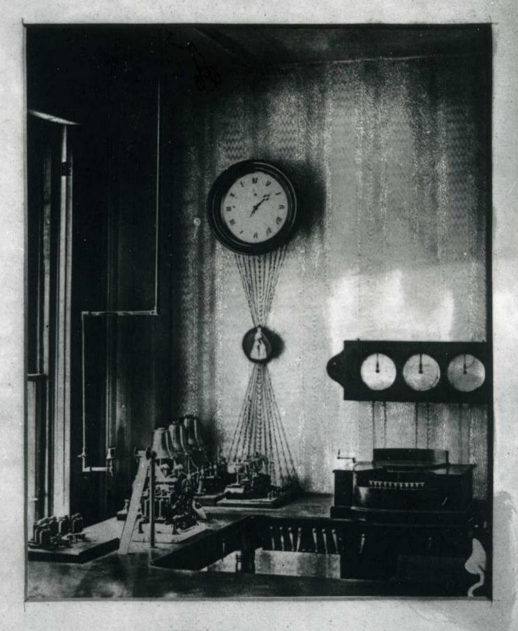
This photograph represents the FIRST ELECTRIC FIRE ALARM APPARATUS ever used. It was located in the City Building, Court Square, placed in service at noon on the 28th day of April, 1852, and gave the first alarm of fire on the following day.
