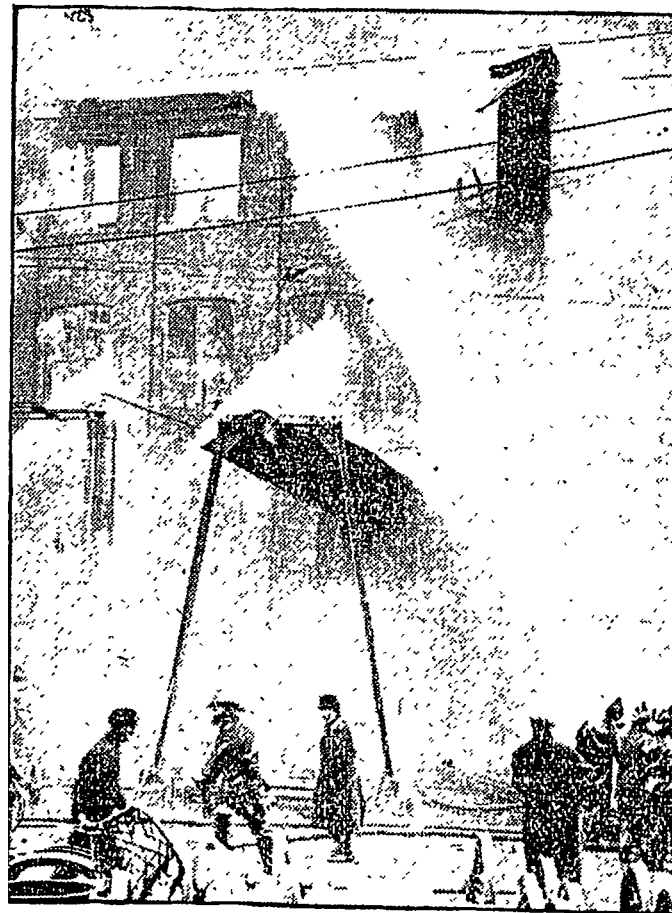
WHERE THE WALLS CRUMBLLED AT FIERCEST CORNER OF THE FIRE.
